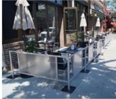
**Figure 4.** This sectional barrier is constructed of metal and plexi-glass.
